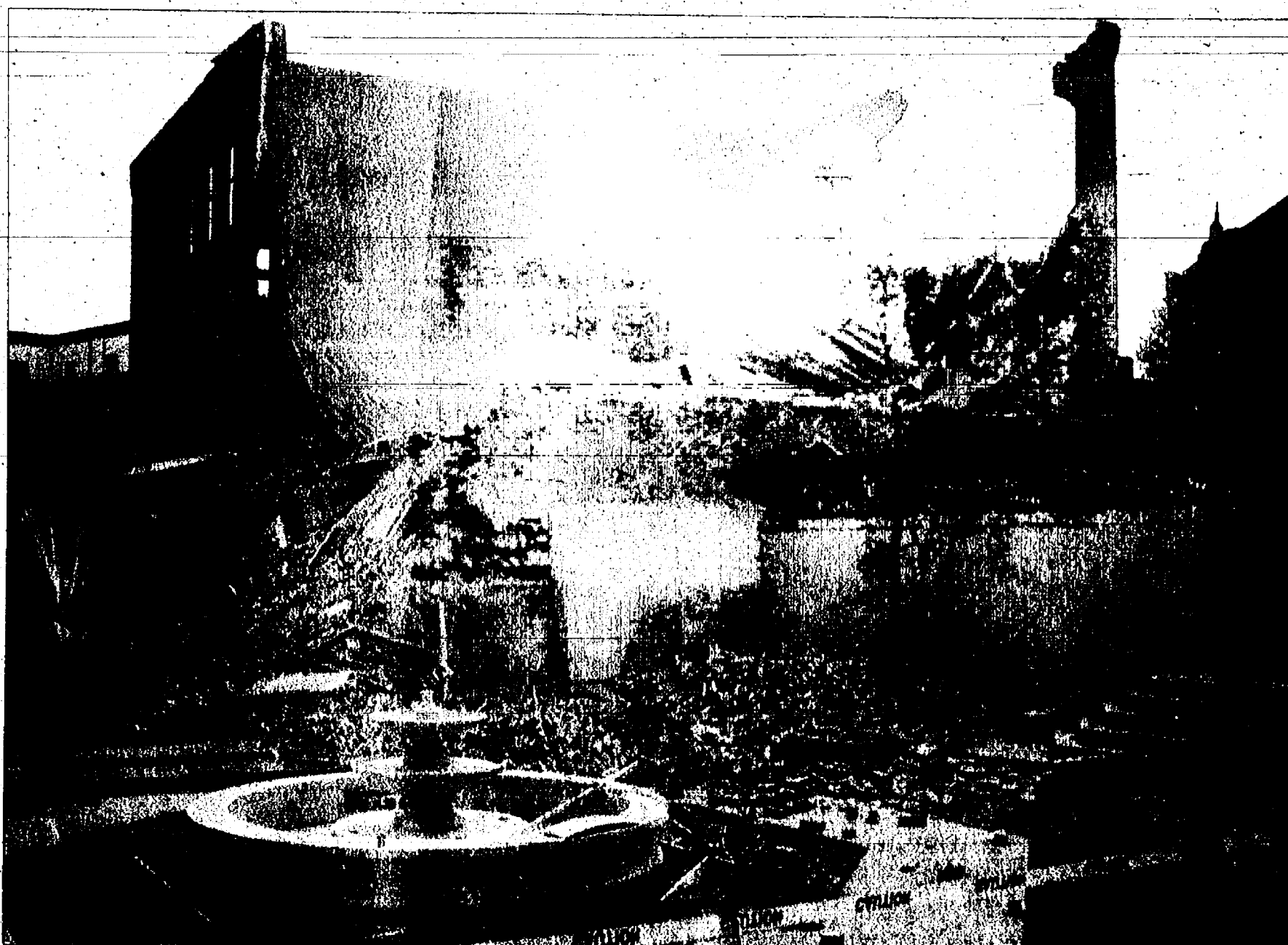
A portion of a former gymnasium building, built as part of Glazier Stove Works in the early 1900s, collapsed last Thursday during renovation work of the Clocktower Complex.
